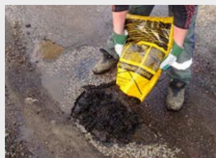
Pour the mix into the cleaned hole straight from the bag.
