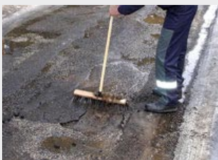
Remove debris, ice or water from the hole in order to improve tacking.
