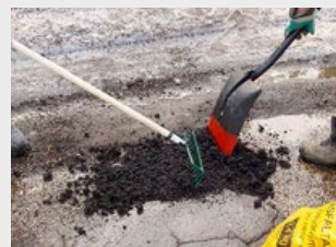
Level out the surface with a spade or a rake, so that the level of the mix remains a little bit above the road surface.
