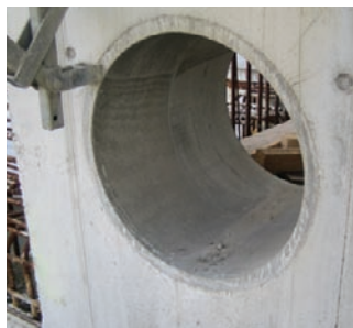
P-LINER Basic 2 FZR 400/300 paigaldus reoveemahutis
