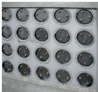
P-LINER Basic FZR 2 100/240 torude tihendamisel
