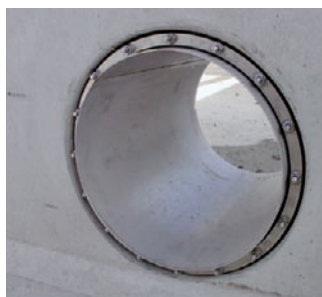
P-PIPE Professional 1 HRD 700-1-1/600 Kinnine tihendi paigaldus
