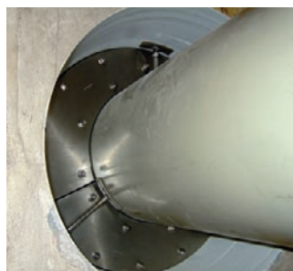
P-PIPE Professional 3 HRD 600-2G-1/420 ex 50 (ekstsentriline tihend, min vahekaugus 50 mm)
